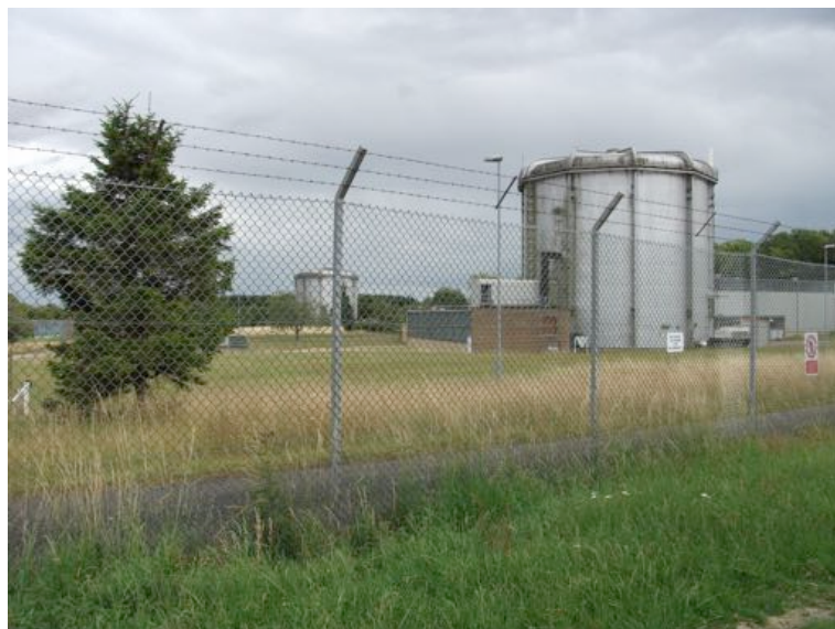
Fig. 6. DIDO and PLUTO – the notices on the fence indicate that it is the boundary of a Nuclear Licensed Site on which trespassing is a criminal offence (author, 2015).
