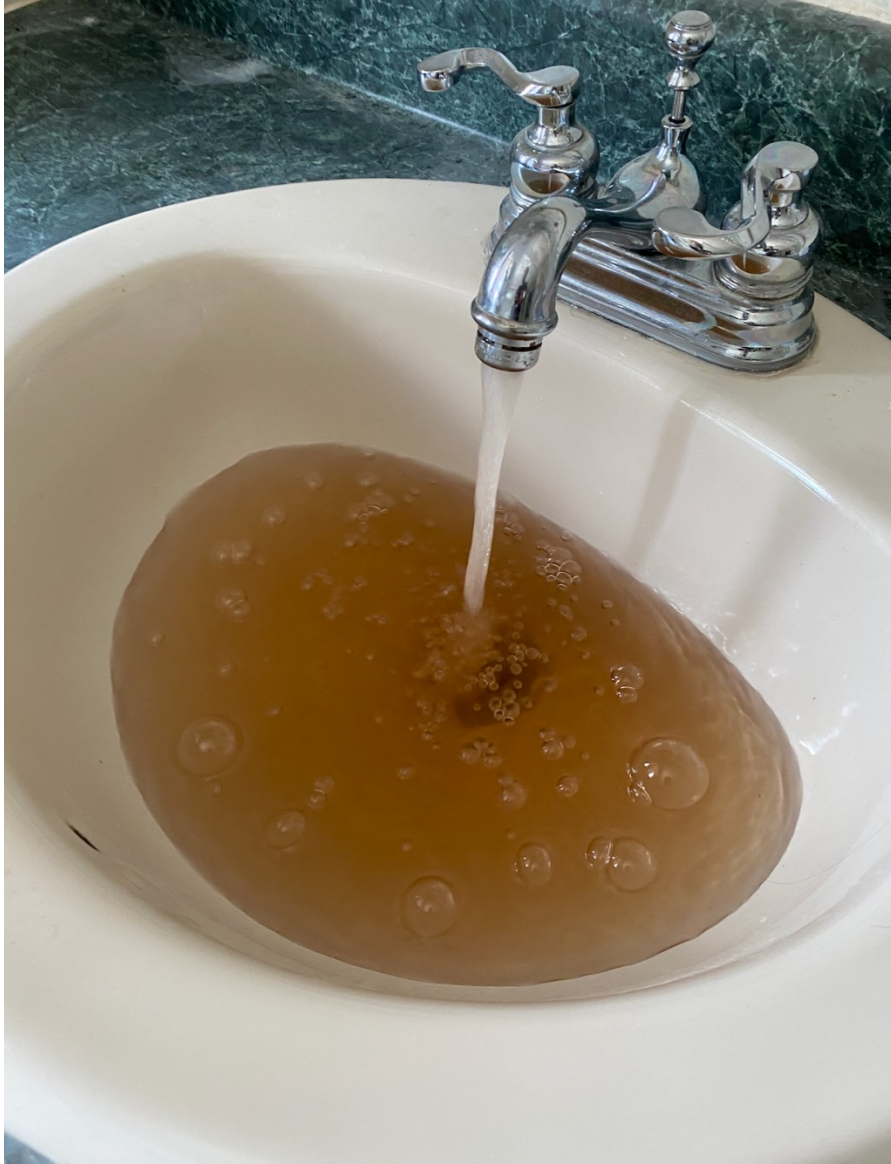
Figure S3: Example of discolored water encountered during flushing on upper floors.
