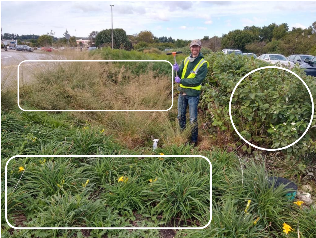
Figure S.2: Picture of a bioretention cell (with co-author LeFevre) with different dominant plants outlined with white shapes as an example of a cell that would be classified as having a “mixed” dominant planting type.
