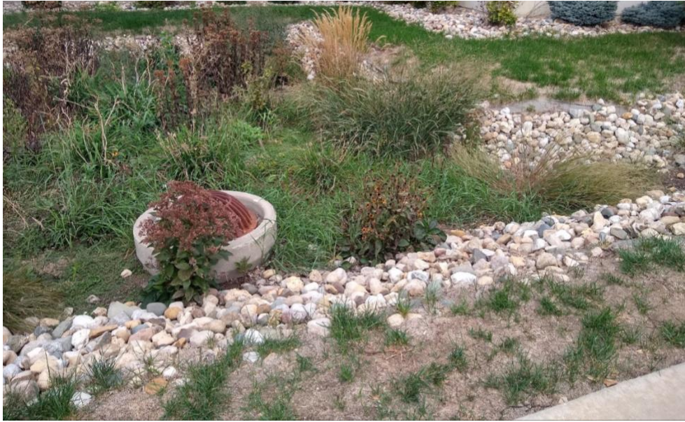
Figure S.1: Picture of a bioretention cell. Bioretention cells are typically depressed areas to receive stormwater, filled with a mostly sandy media for quick infiltration, and often vegetated. This bioretention cell has an overflow drain structure (the circular grate).
