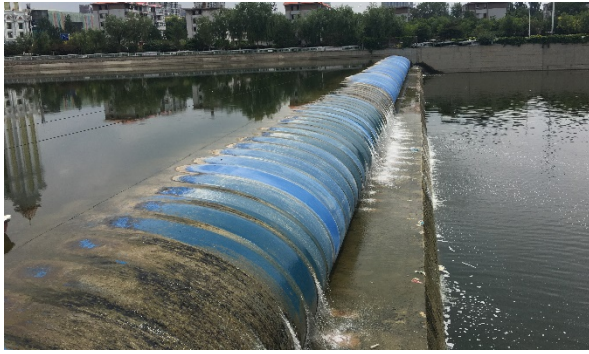
Rubber dam (Lower-reach)
