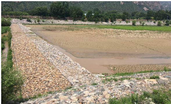
Sand trapping dam (Lower-reach)
