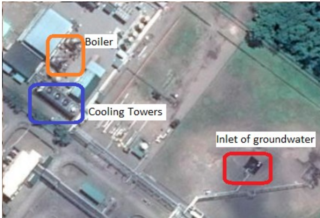
Figure 6. Example of the infrastructure seen in Satellite Images of groundwater-fed cooling towers.
