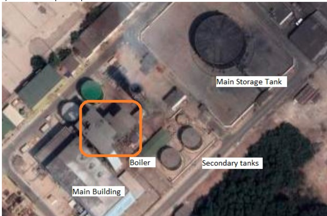
d) Biomass power plants
