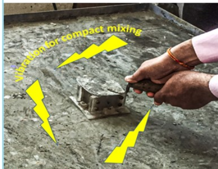
Homogenize and compaction through vibration
