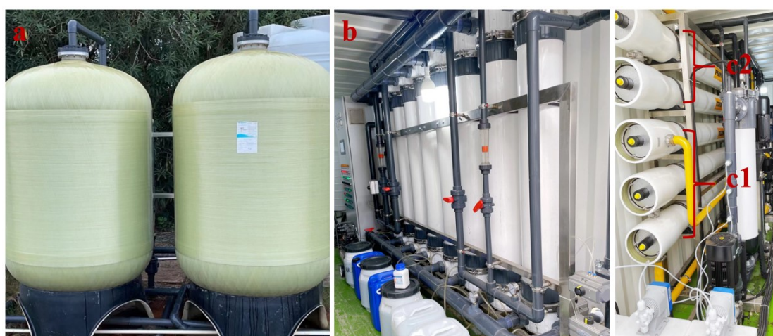
a: Sand filter tank, b: UF membrane module, c1: first stage RO membrane module, c2: second stage RO membrane module
